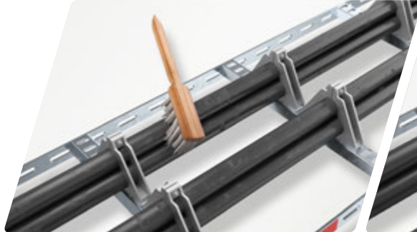
1. Clean dust and dirt from cables/cable support structures.
